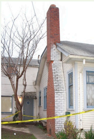
Chimney damage
