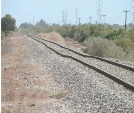
Train tracks were bent by ground movement
