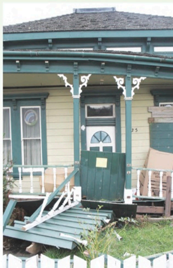
Cripple wall failure
