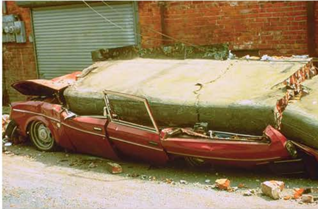
Unreinforced masonry damage
