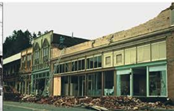
Unreinforced masonry damage
