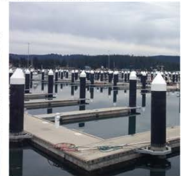
Crescent City's harbor was rebuilt. The new piers will withstand a repeat of 2011. They won't survive a Cascadia tsunami.
