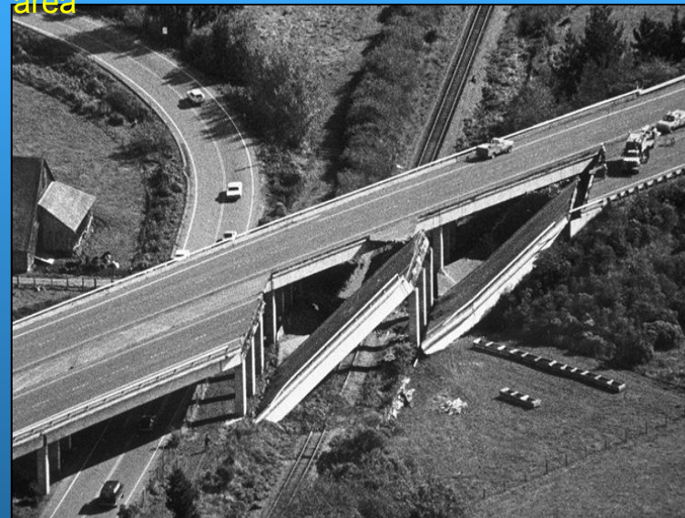
Thompkins Hill overpass damage from the 1980 Trinidad earthquake
