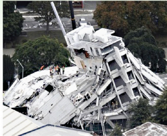
The Pyne Gould Company Building is a six-story reinforced concrete structure built in the 1960s. Twelve people died in the collapse of this building.
