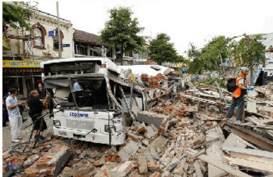
Strong shaking caused damage beyond building collapse. Bricks and other debris were thrown into the street, crushing people and objects like this bus.
