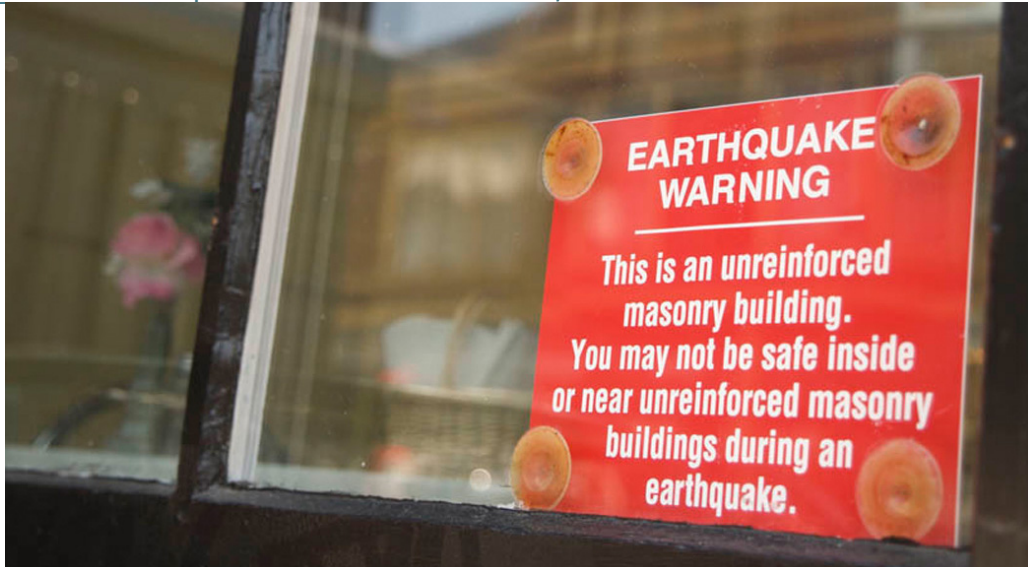
A sign at the entrance to a brick building in Eureka's Old Town warning that it could collapse during an earthquake.
