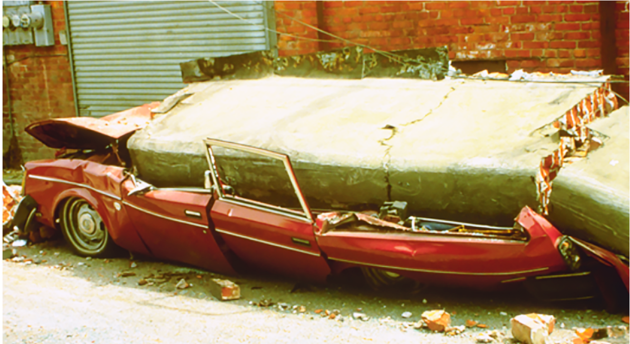
Car crushed by the toppled back parapet wall of the Valley Grocery in Ferndale during the 1992 M7.2 mainshock.
