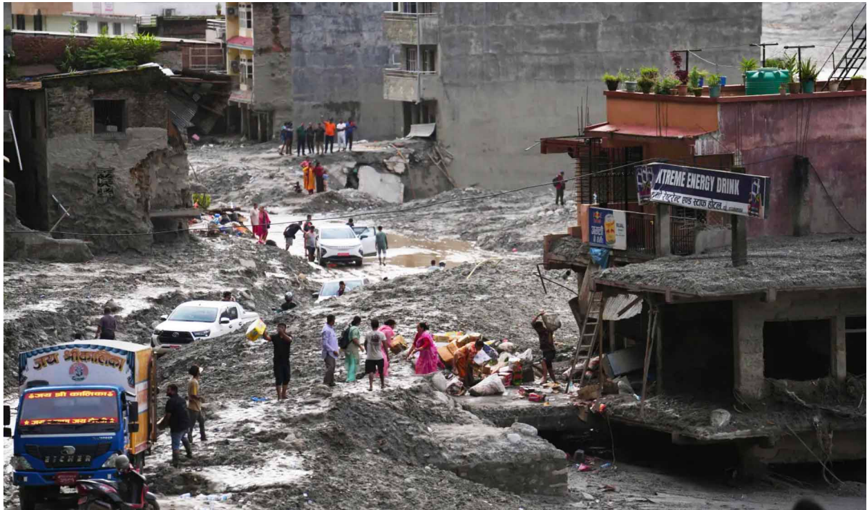
People salvage their belongings from a building damaged by flash flooding in Nuwakot district of Nepal, Tuesday, Sept. 1, 2026. (AP Photo/Rajesh Kumar Singh)
