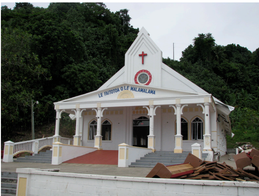
Church in Poloa withstood the tsunami but was flooded and filled with debris.
