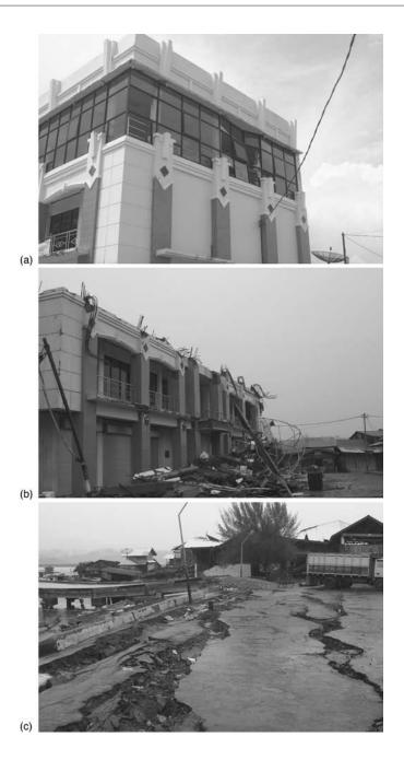
**Figure 2.** Structural damage on Simeulue after the 26 December and 28 March earthquakes. (a) Clearly visible (albeit minimal) structural damage sustained in a new market building in the capital of Sinabang after the December event. (b) The same building after the March event; the third floor has been sheared off. (c) Evidence of liquefaction at the Sinabang harbor after the March event.
